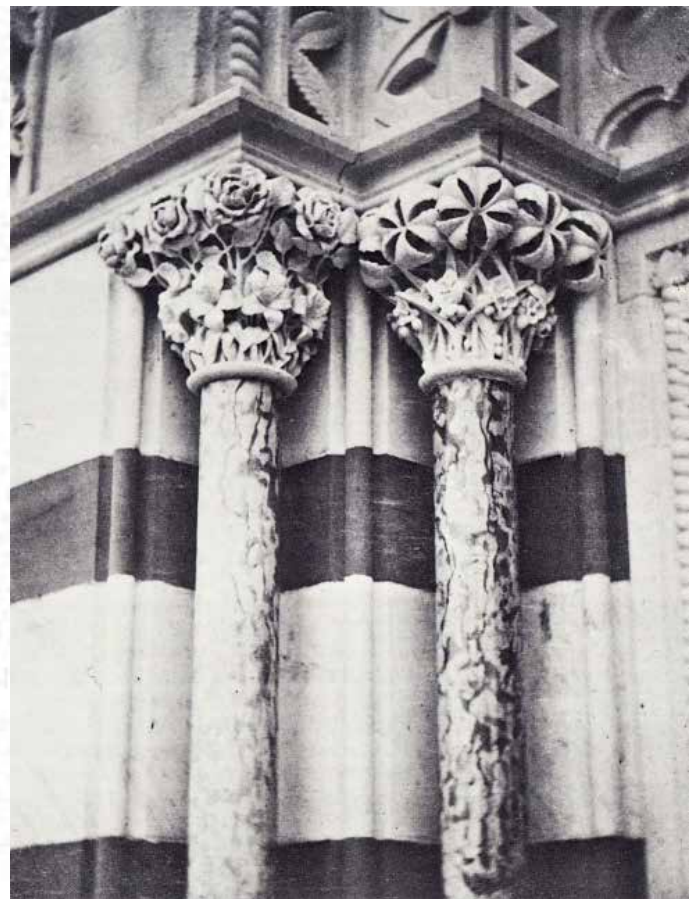
Figure 4. National Academy of Design 4th Avenue Entrance Columns
